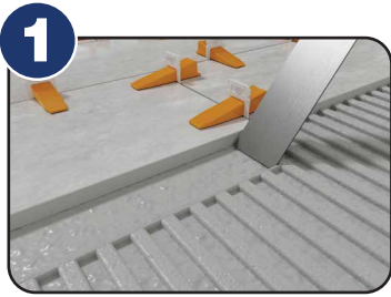
1 Clean excess thinset along tile edge
