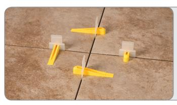
**LEVEL:** Anchor adjusts to the tiles so they remain level throughout the installation
