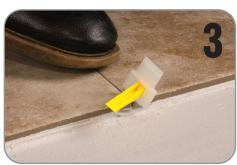
Once mortar has set, simply kick the clips to snap off at the specially designated break-points. Save wedges for future use.
