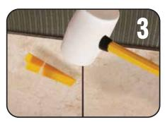
Once mortar has set, simply tap the clips with a non-marring rubber mallet to snap off at the specially designated break-points. Save wedges for future use.
