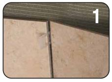
Slide two clips under the tile and into the mortar approximately 2" from each end of the tile. Place the second tile.
