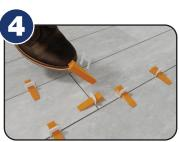
Once the mortar sets, remove in direction of grout line within 24 hours
